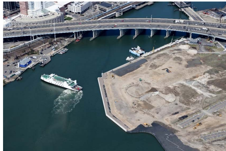
RACE was nationally recognized by the American Council of Engineering Companies (ACEC) for its innovative approach to the Steelpointe Harbor Waterfront Project in Bridgeport, CT
